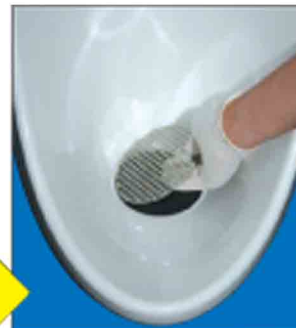
Insert new filter or cleaned filter
