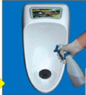
Interior cleaning: Spray with BIOX cleaner of Urimat
